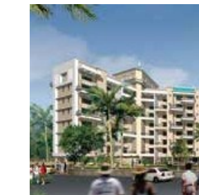
REGENCY ROSELAND Talegaon, Pune
