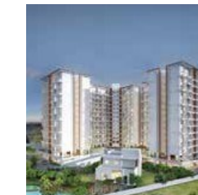
REGENCY ORION Baner Pune
